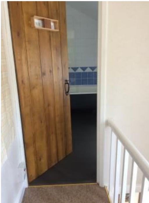
Bathroom at top of stairs at the end of the landing with level access from the single bedroom. Door width is 72 cms.
